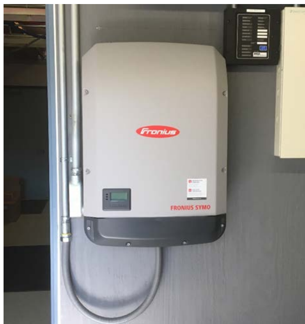
Figure 16 - Inverter
